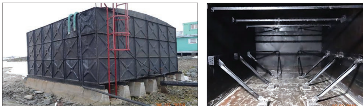
Figure 2. The decommissioned old fuel tank HST-150, outside and inside view
